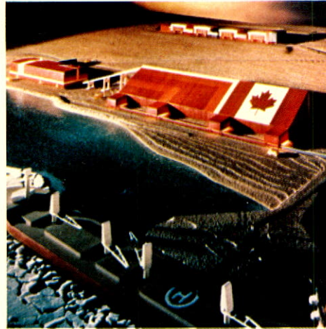
Model of the Polaris Mine, N.W.T., showing dock (foreground), processing plant, concentrate storage building (centre) and accommodation complex (background).
