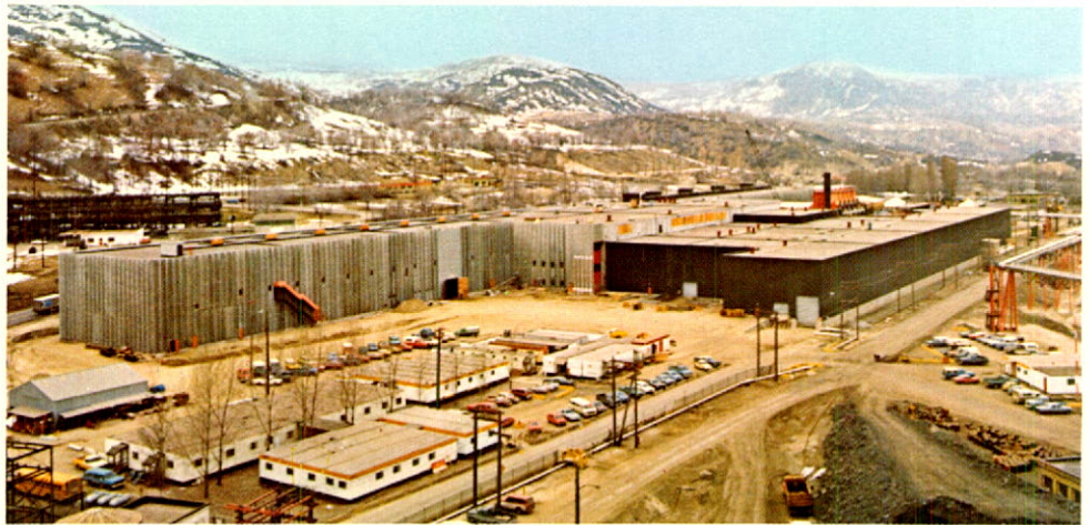
The $210 million zinc electrolytic and melting plant at Trail will be partially operational in 1981.
