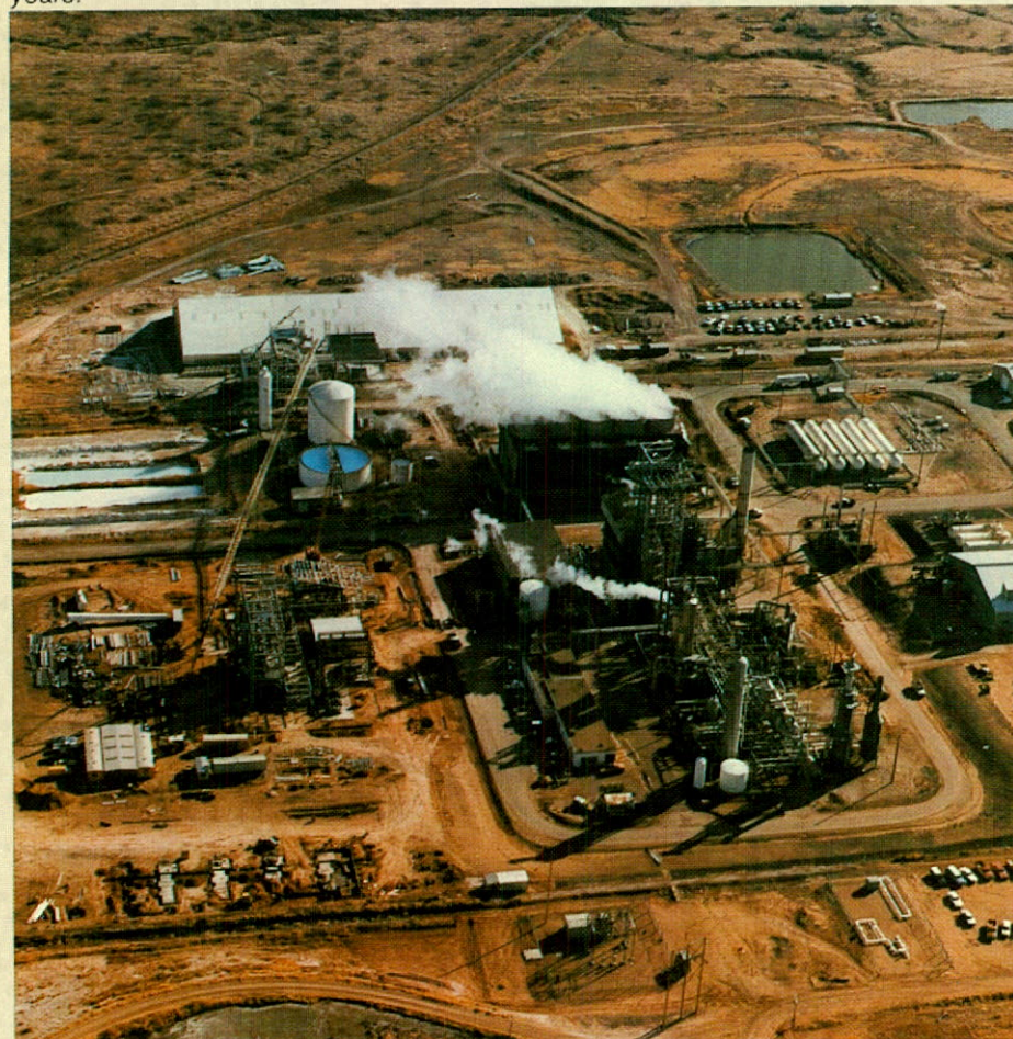
A new urea plant (left centre) adjacent to Cominco American's ammonia plant at Borger, Texas, will use 48,000 tons of ammonia annually in the production of 85,000 tons of urea.
