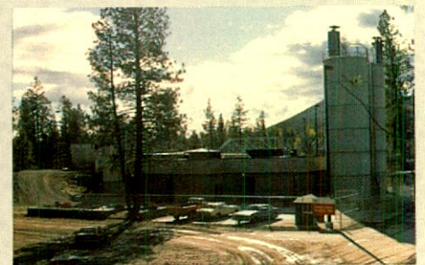
$10 million Drainage Water Treatment Plant at Kimberley removes metallics from drainage water out of the Sullivan mine and concentrator tailing ponds and discharges clear water into the Kootenay River system.
