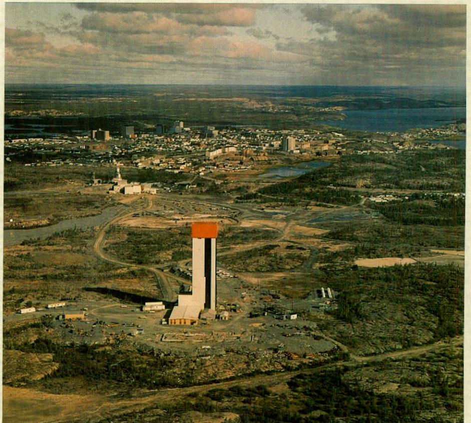
The 250 foot headframe of the Con gold mine is becoming a familiar landmark in Canada's North. Housing the hoisting mechanism for the 5,400 foot deep Robertson shaft, it provides an impressive addition to the skyline of the City of Yellowknife.
