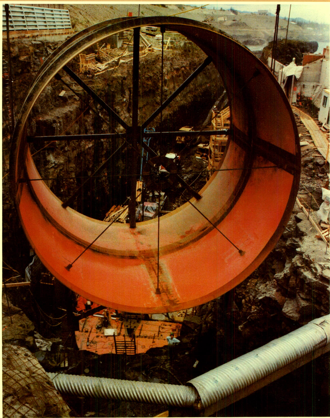
BELOW: Penstock liner and tailrace excavation for North- ern Canada Power Commission project in Whitehorse, Yukon.
