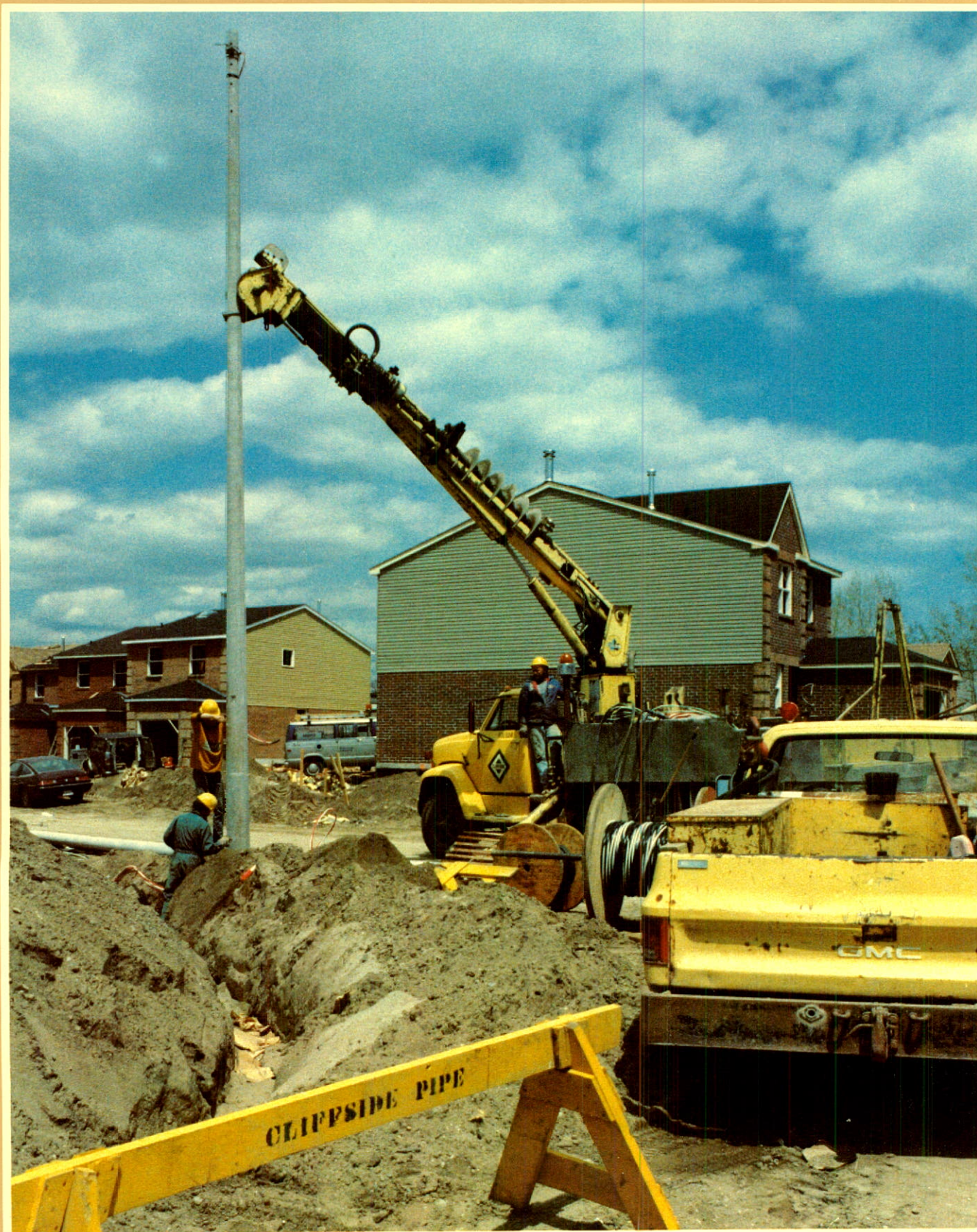
BELOW: Cliffside crew installing streetlight poles as part of redevelopment program near downtown Toronto.
