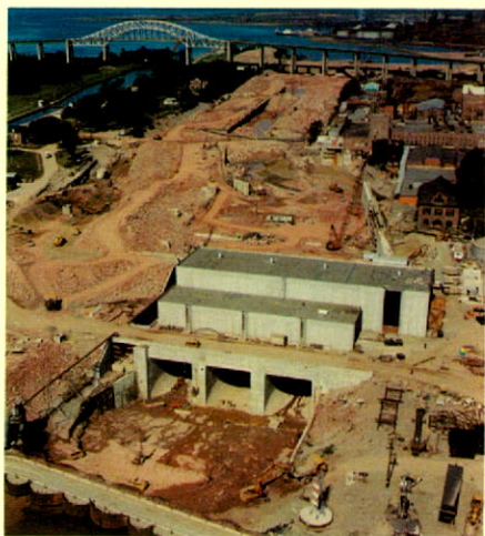
ABOVE: Three-unit horizontal bulb turbine generating station in Sault Ste. Marie, Ontario. The Sault Ste. Marie international bridge in the background was completed by Pitts in the early 1960's.
