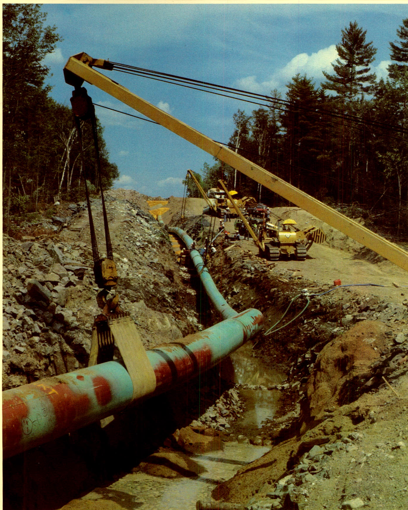
BELOW: Lowering in on TransCanada PipeLines' "North Bay Shortcut" project. Fifty-three pipelayers were required on this job.
