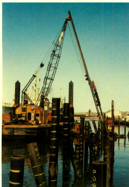
ABOVE: Manitowoc 3900 working off "Canadian Jubilee" drives pile for Canadian National Railway's ship repair facility in St. John's, Newfoundland.
