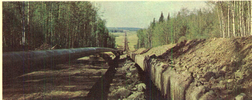
Pipeline looping to accommodate increased production at Minnehik-Buck Lake Gas Plant
