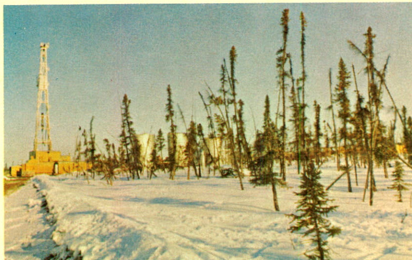
Winter drilling operations, Northwest Territories
