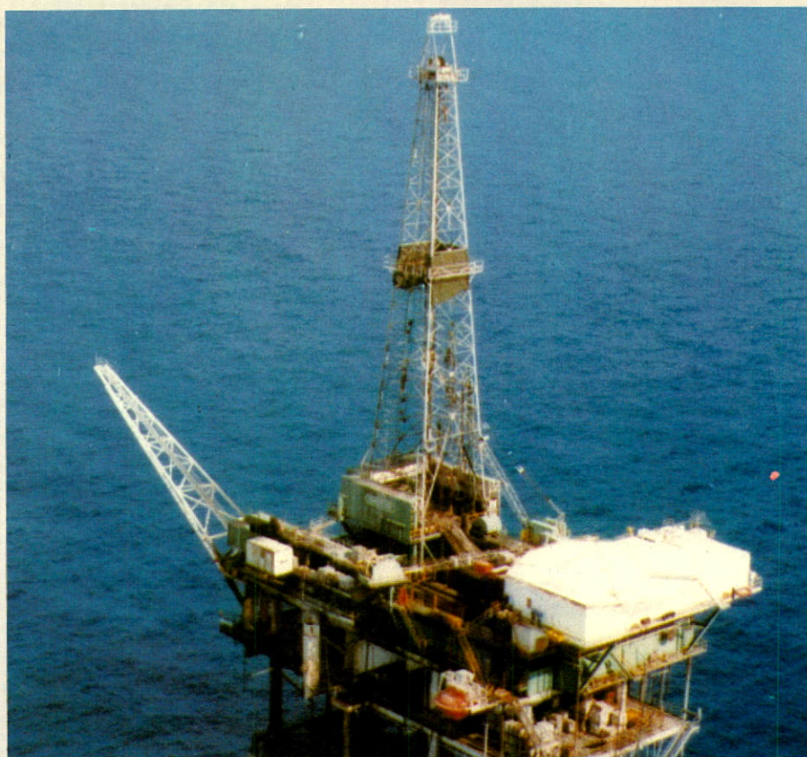
Permanent Drilling and Production Platform.
