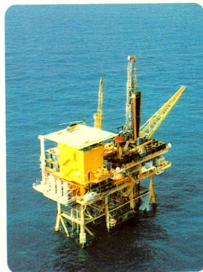
Permanent Drilling and Production Platform in the High Island area, offshore Texas.
