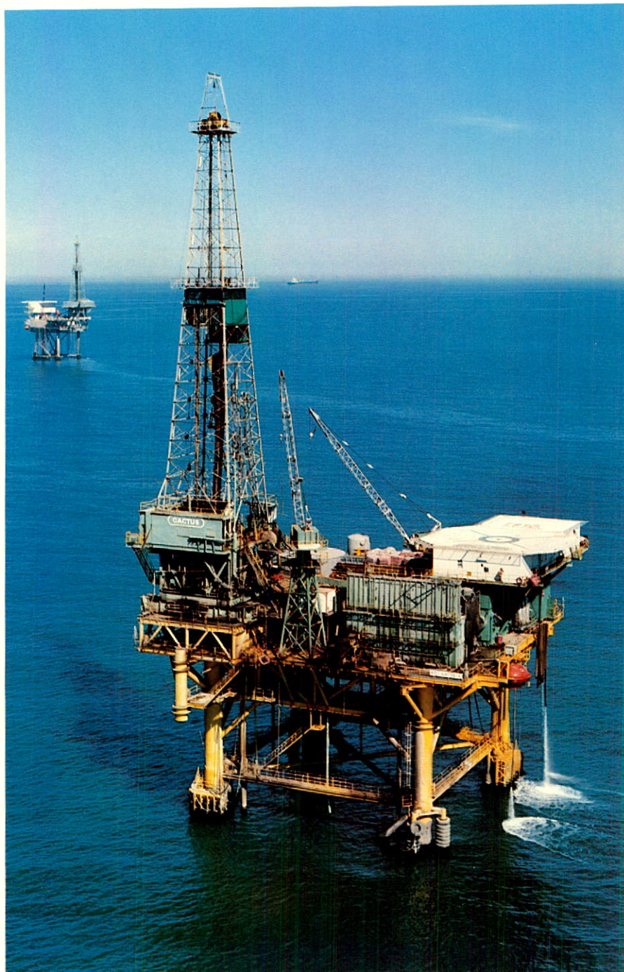
Drilling and production platform at South Pass Block 78 in the United States Gulf Coast.
