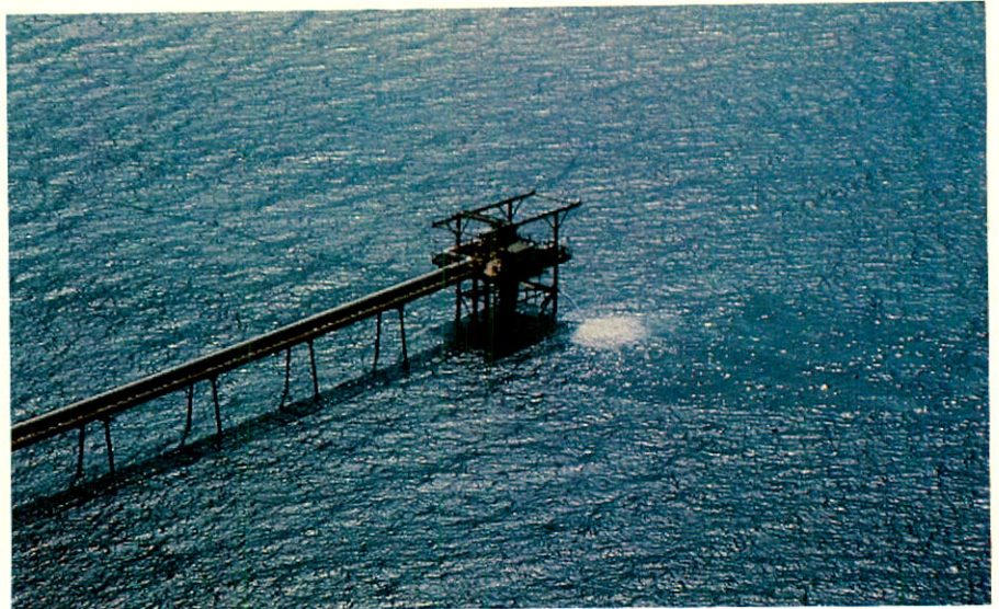
Seawater intake facilities at Talara, Peru.
