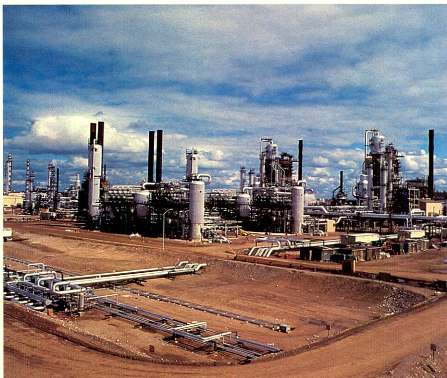
Syncrude plant near Fort McMurray, Alberta.
