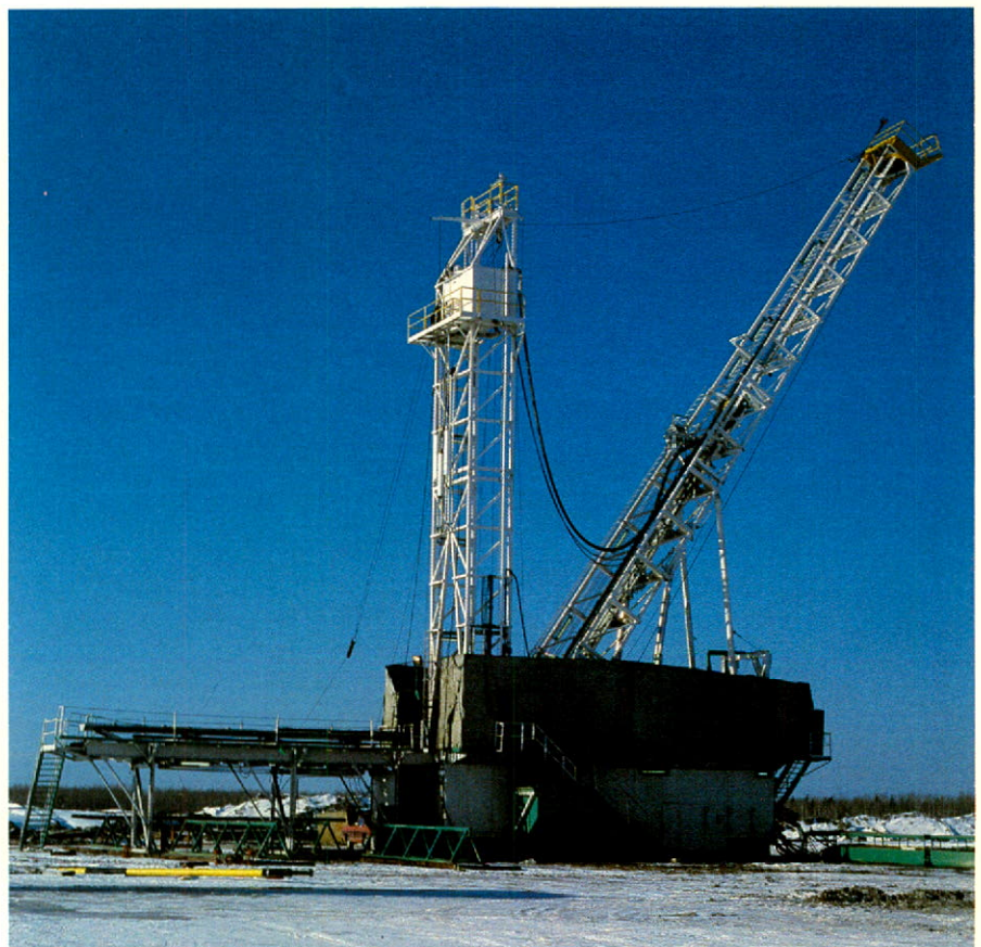
Slant drilling at Manatokan steamflood pilot project in Alberta.
