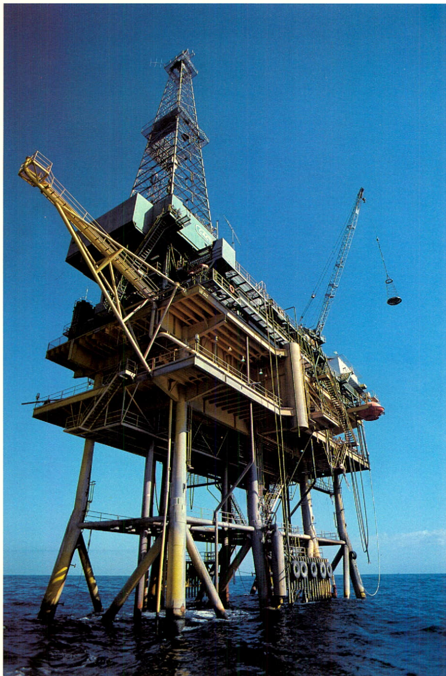
Drilling and production platform in the United States Gulf Coast.
