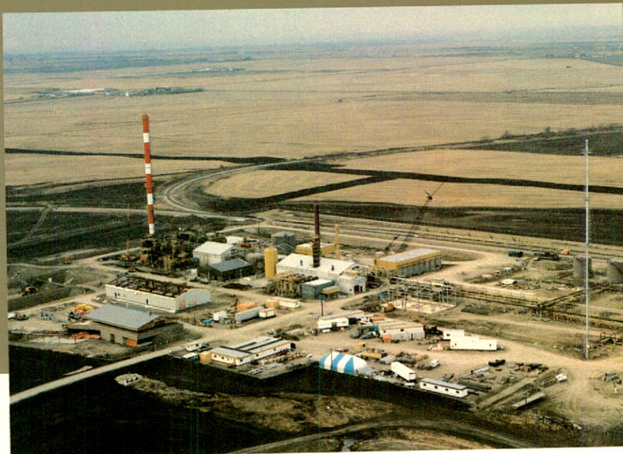
Mazeppa gas plant, south of Calgary, under construction.
