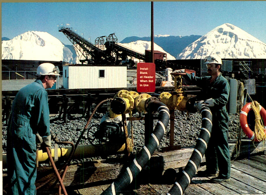
Loading caustic product onto barge at North Vancouver plant.
