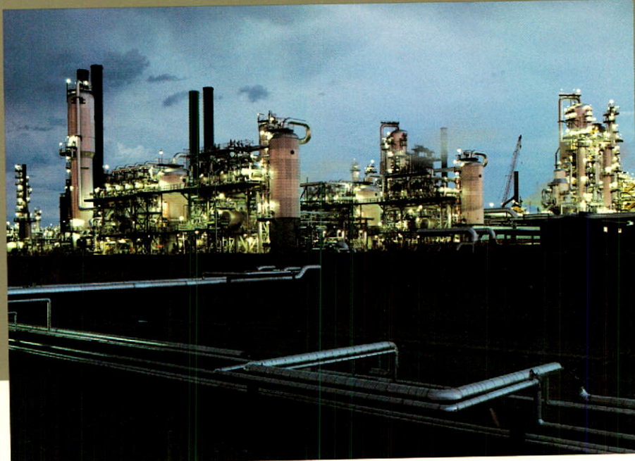
Syncrude plant near Fort McMurray, Alberta.
