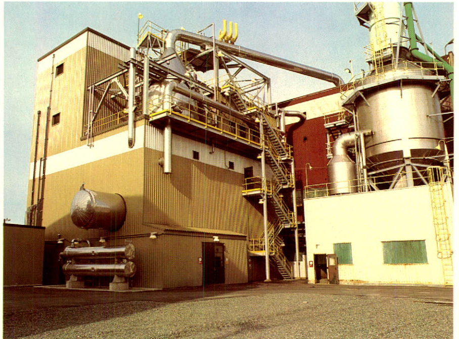
New caustic processing facilities at the North Vancouver chlor-alkali plant.
