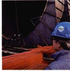
Dominion Bridge-built module for vehicular tunnel beneath Baltimore harbour.
