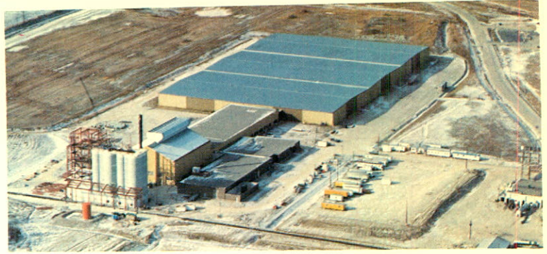
The new Milton, Ontario plant now under construction
