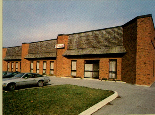
The PLAX plant in Brampton, Ontario, is one of three PLAX INC. plants.
