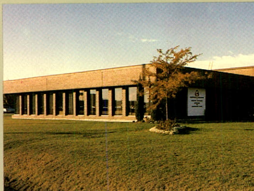
The Portion Packaging plant in Rexdale, Ontario, produces a wide range of thermoformed plastic packaging.
