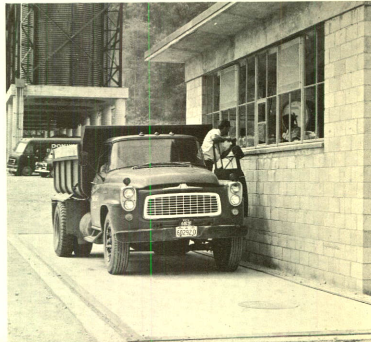
Installation of a Howe Motor Truck Scale that weighs trucks leaving the new Dufferin Quarry, Milton, Ont. This scale is engineered to give accurate and speedy weighing for long continuous service. The all-steel construction insures maximum strength with minimum weight factor.
