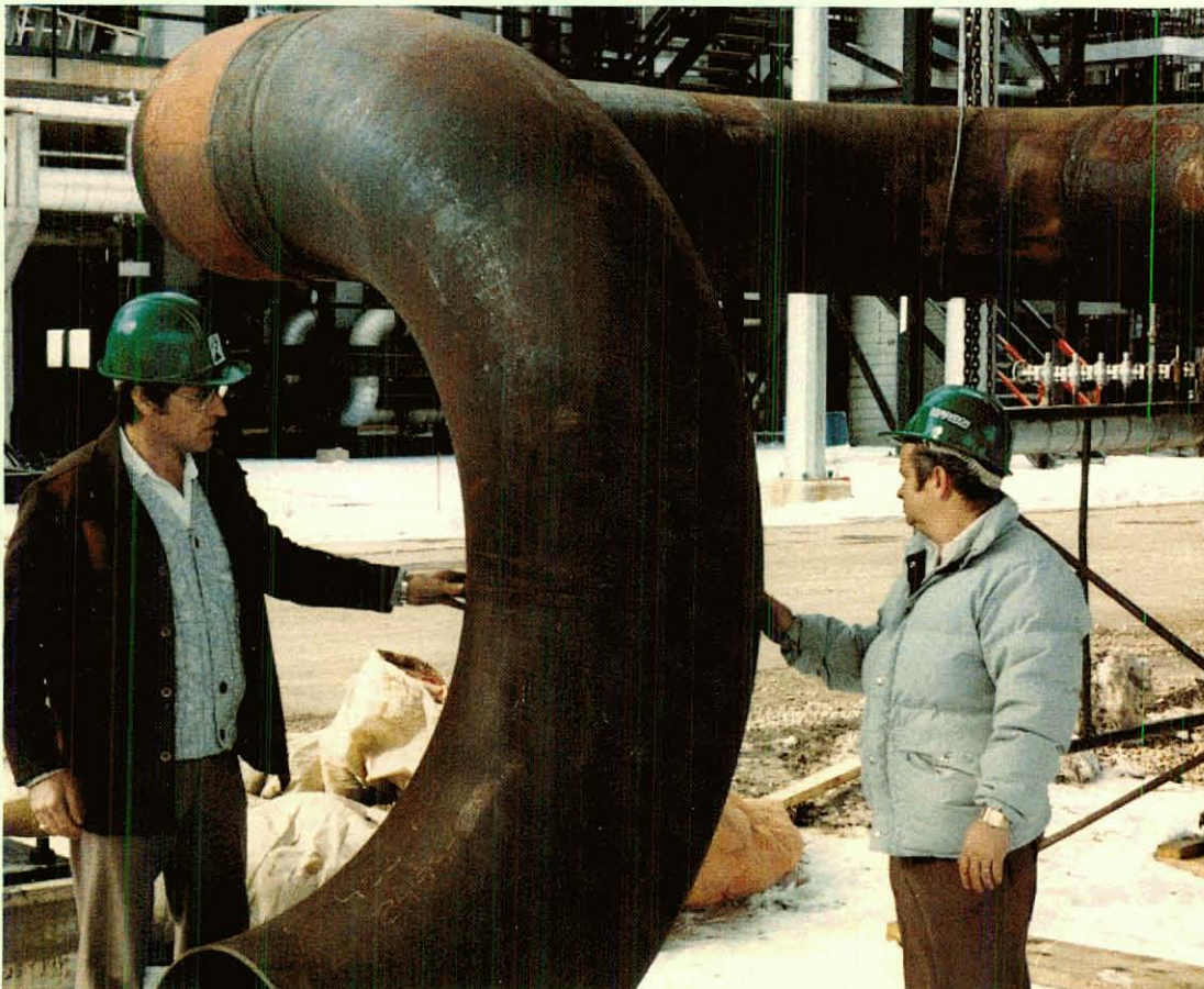
Inspection of an 18" steam line being rigged for high line at Imperial Oil Limited's Strathcona Refinery, Edmonton, Alberta.
