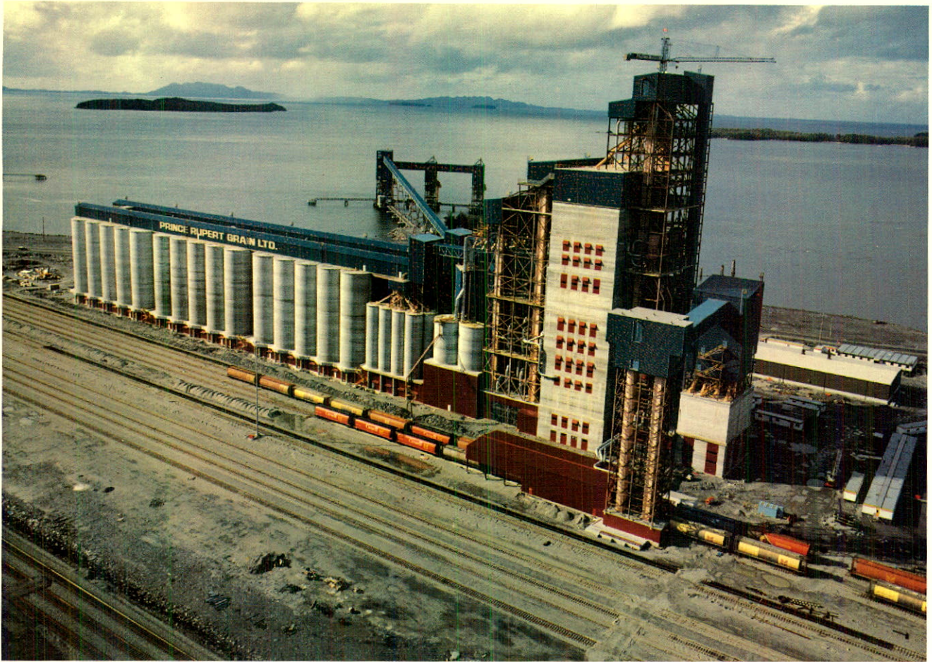
The Prince Rupert Grain Terminal on Ridley Island, British Columbia will store up to 200,000 tonnes of grain in its 92 silos.
