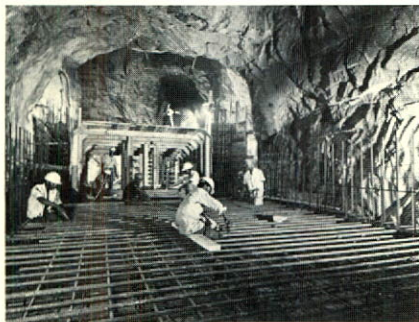
Reinforcement in draft tube
