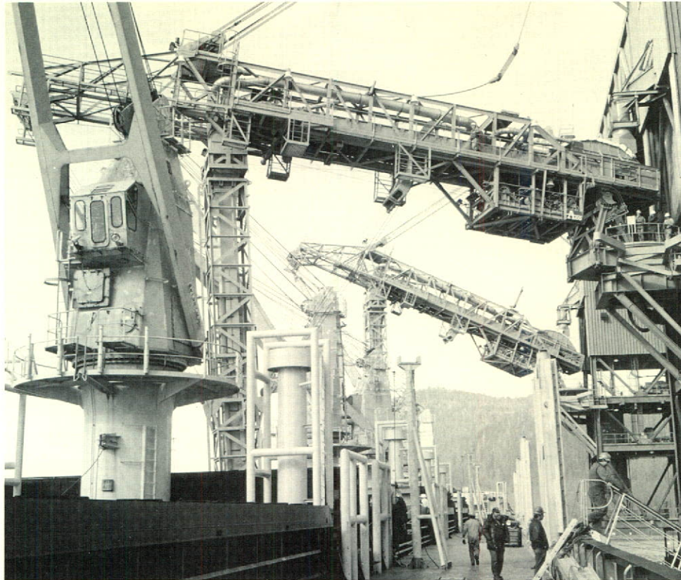
Ship Loading Facility, Prince Rupert Grain Terminal, British Columbia
