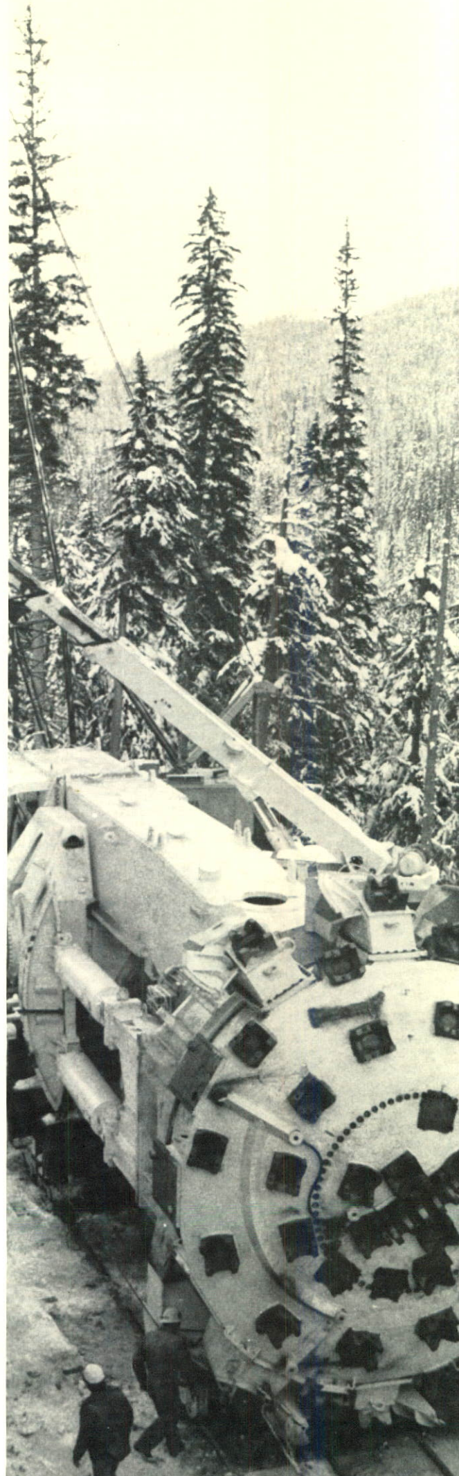
Tunnel Boring Machine, Rogers Pass, British Columbia
