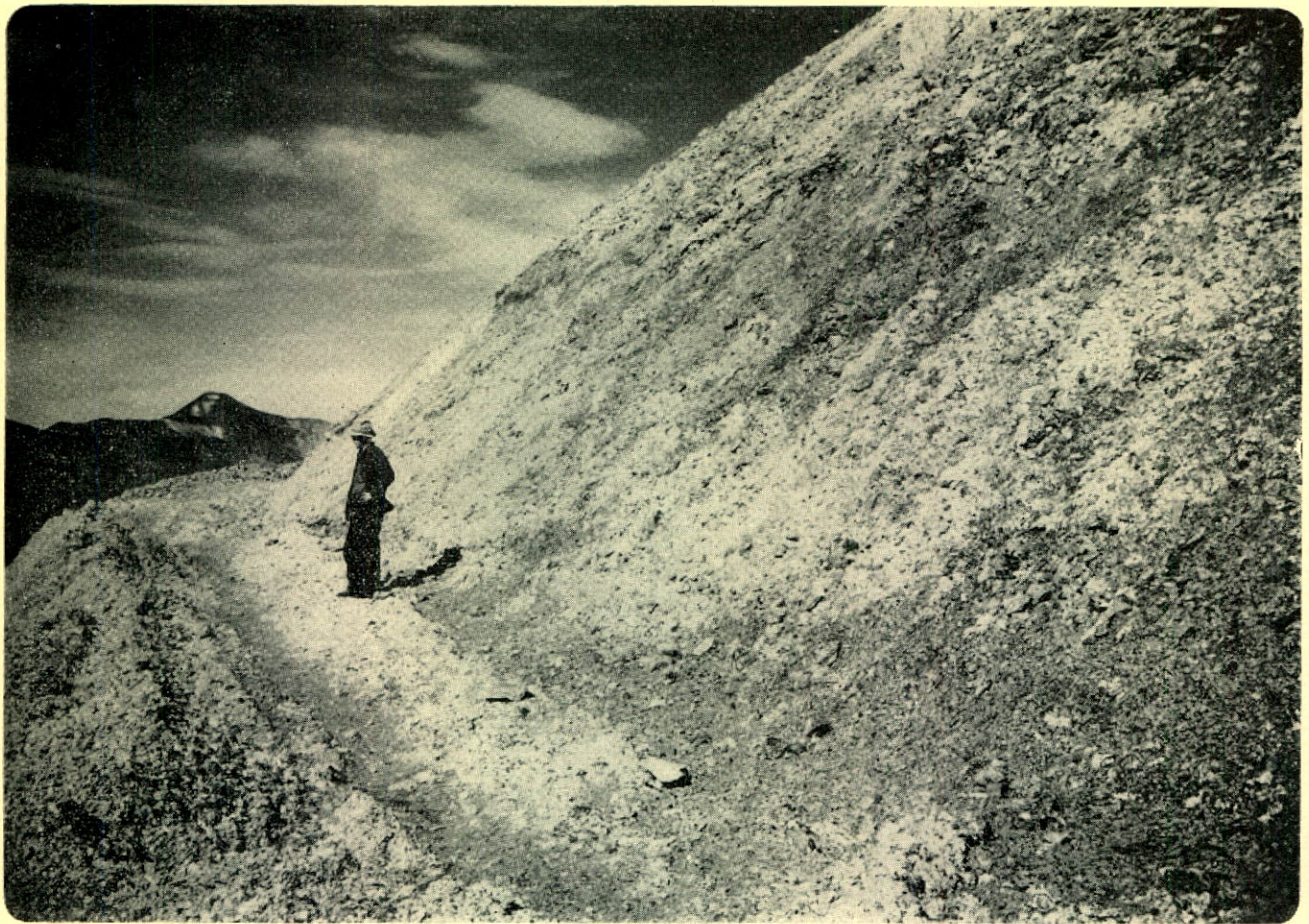
Road cut through asbestos talus near top of showing, western slope of mountain.
