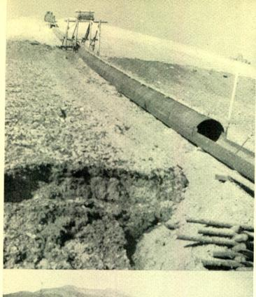
Upper portion of steel chute used to transfer ore from the mine to the truck loading bins.
