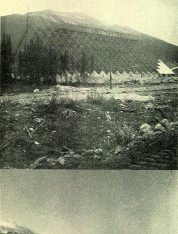
Forty thousand ton capacity dry rock storage building illustrating type of construction.
