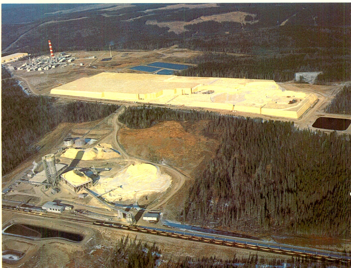
The sour gas processing plant and sulphur block at Ram River with the prilling tower and sulphur handling facilities in the foreground.
