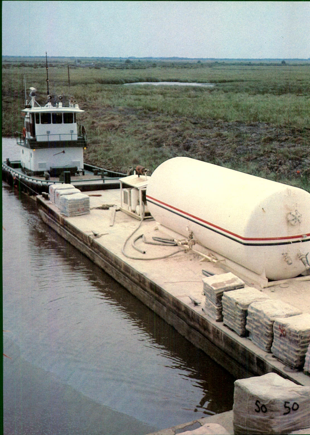
A barge pulls equipment to do well servicing work on Canterra's discovery well in the North Deep Lake field in Cameron Parish, Louisiana.
