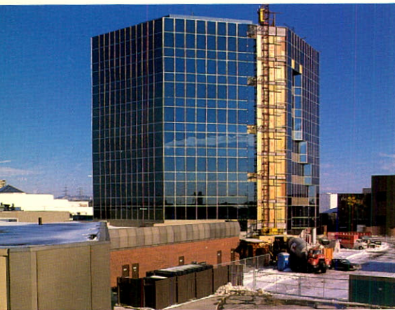
Place Vertu, Montreal - a 100,000 square foot office tower under construction
