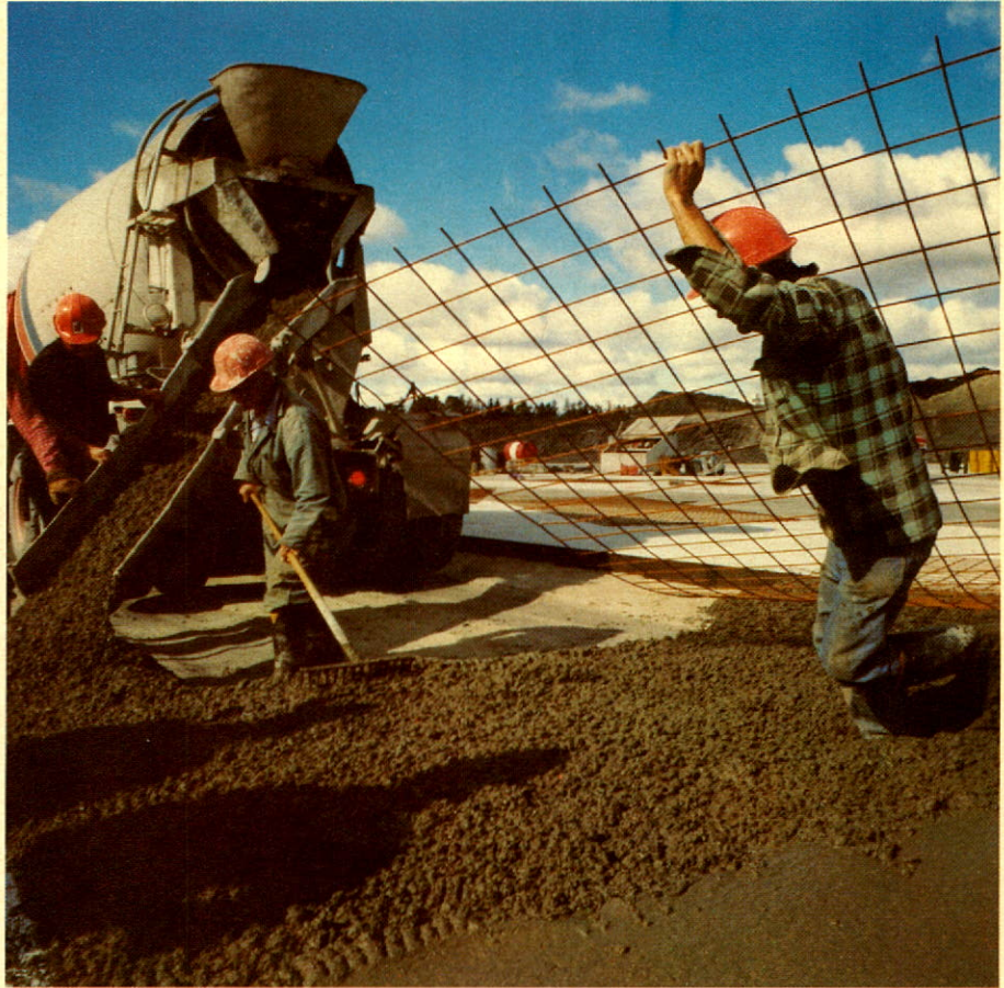
Construction of concrete pad for coal storage, Mississauga plant.
