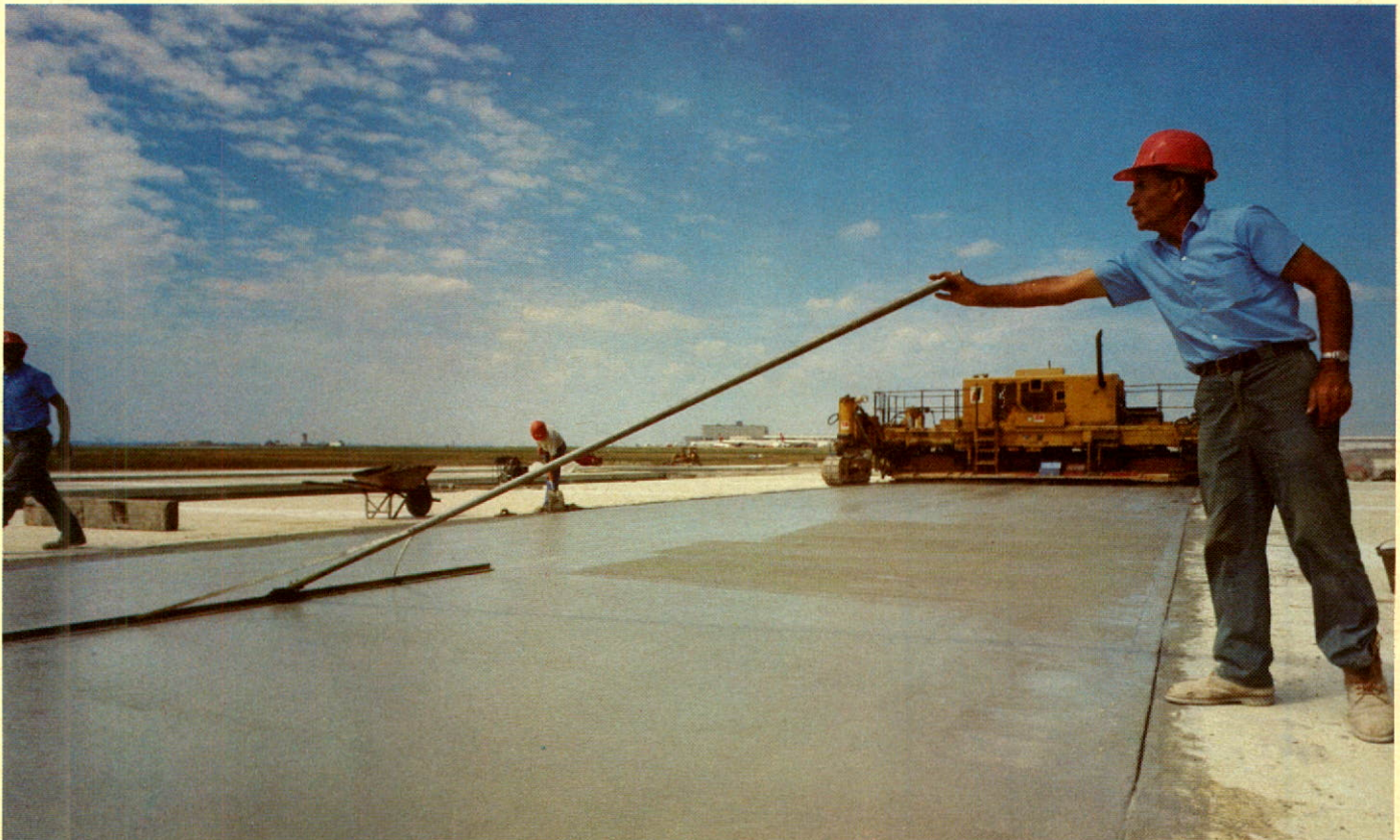
Construction of approach runway to new Wardair hangar, Toronto International Airport.
