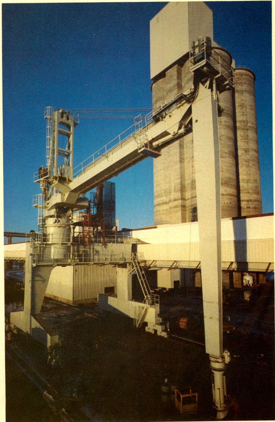
Marine Cement Terminal in Duluth with the "Siwertell" unloading system.
