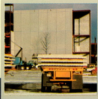
The buildings on the Crossgates Shopping Mall site at Albany, N.Y. used precast façade panels with cement supplied by I.C.C.
