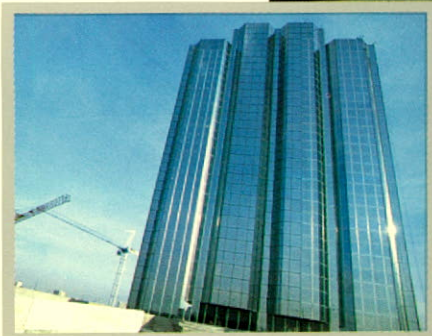
Utilization of concrete supplied by Dufferin Concrete Products in the construction of the Consilium Development, a prestigious new office complex in Scarborough, Ont.
