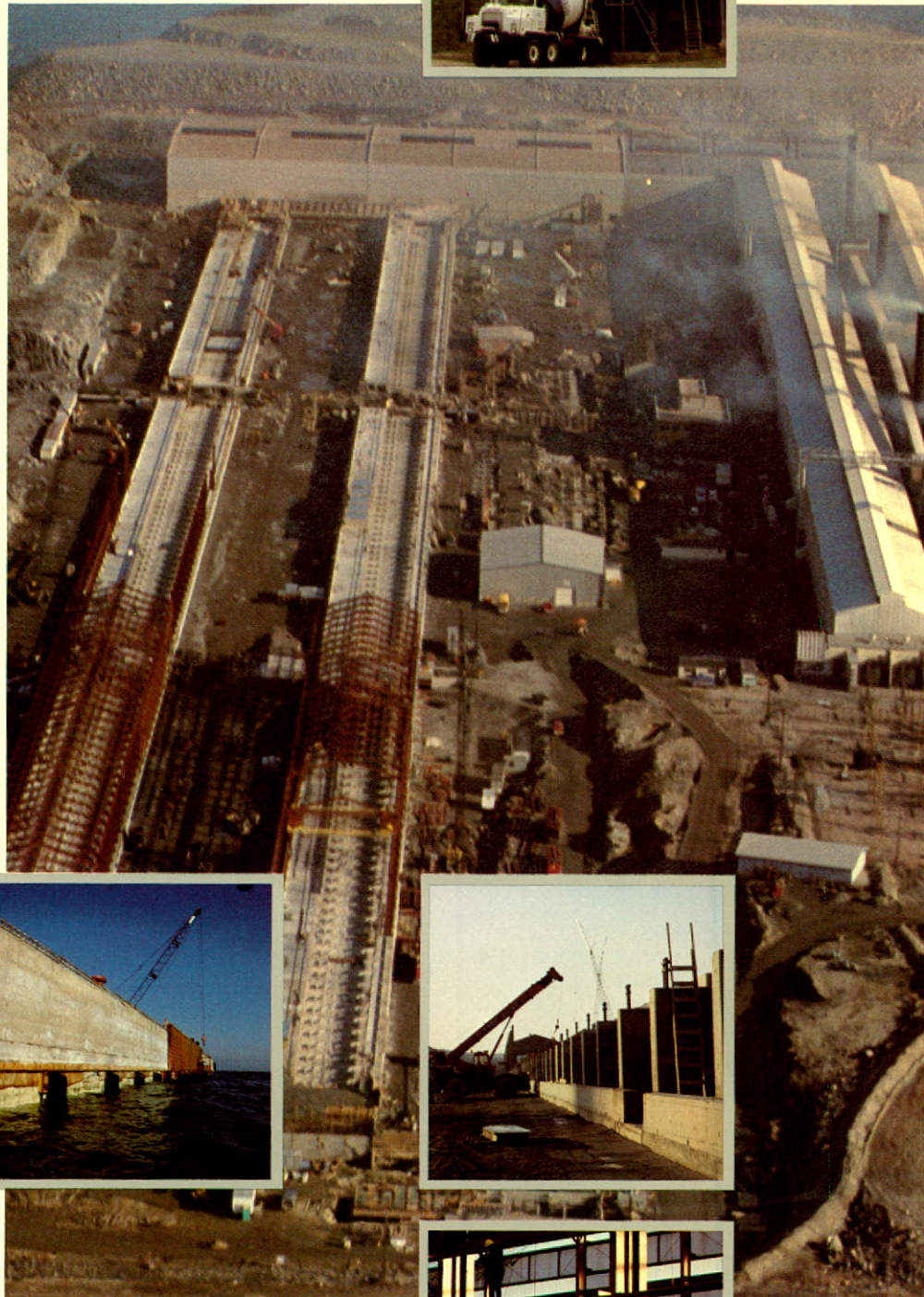
Expansion of the Canadian Reynolds Metal Co. Ltd. plant at Baie Comeau. Over 65,000 cubic metres of concrete supplied by Béton Manicouagan are needed for the construction of the two pot rooms D1 and D2.
