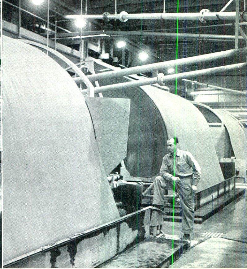
TAILINGS DISCHARGING FROM MILL FILTERS
