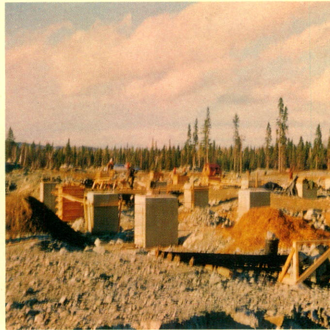
Above: Mill foundations readied for steel erection.
