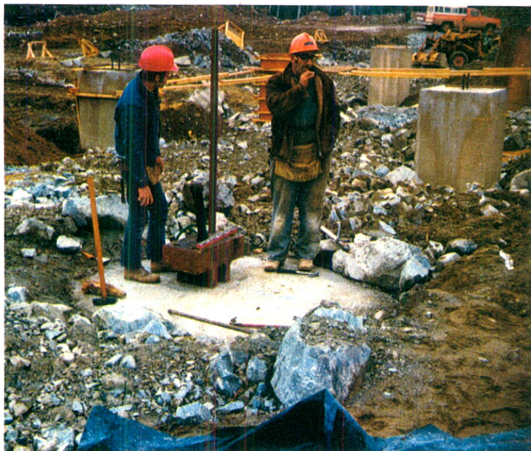
Above: Placing of 20 foot cables to anchor mill building.
