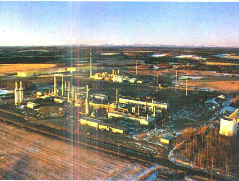
The gas plant now under construction in the Strachan-Ricinus area will be similar to this completed plant in the same vicinity. U.B.R.'s production from the new plant will be sold to Trans-Canada Pipelines Limited under a 25-year sales contract.
