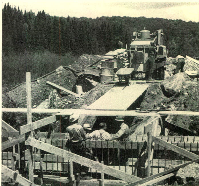
Building one of the many steel-reinforced culverts on the Trenché road. Culverts had to be specially strong to carry the vast quantities of material and extremely heavy equipment.
