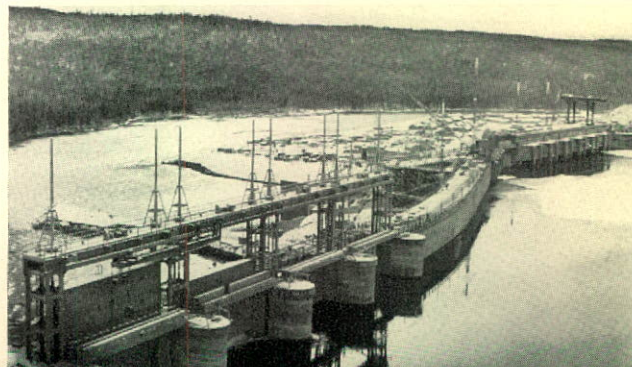
The main dam rises foot by foot from the dry river bed. In the background are the by-pass and gatehouse sections and the steel framework of the powerhouse.
