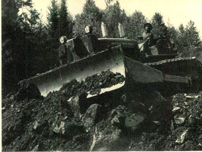
A monster bulldozer at work on a difficult section of the road. Many such huge machines and a fleet of trucks were needed for the job.
