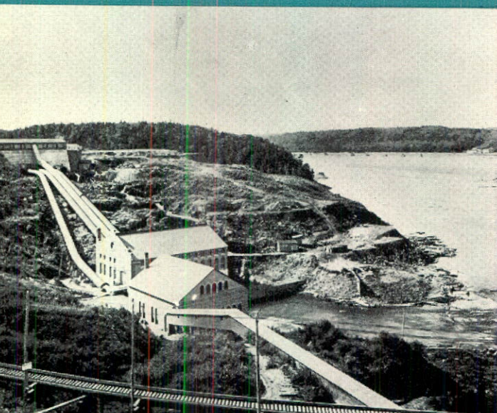
Power developments at Shawinigan Falls in 1903 — installed capacity 10,000 hp.
