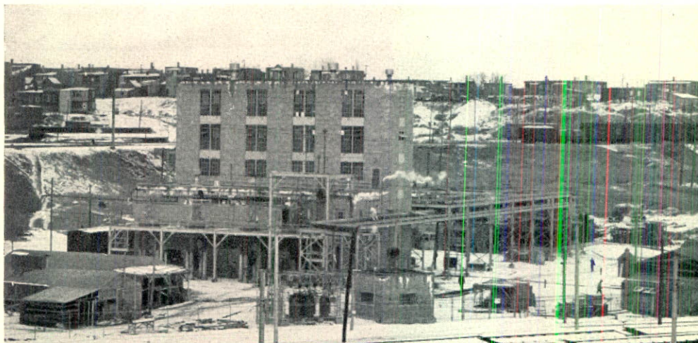
The new Dioctyl Phthalate Plant of Canadian Resins and Chemicals Limited.
