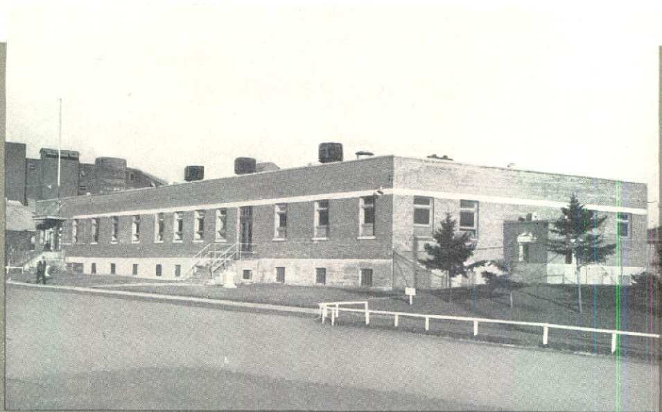
Welfare Building at the Carbide Division
