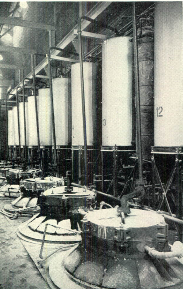
Interior view of one of the Chemicals Company's manufacturing plants.
