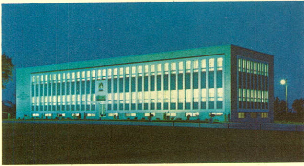
The Company's new Valleyfield service building, officially opened in June 1961.
