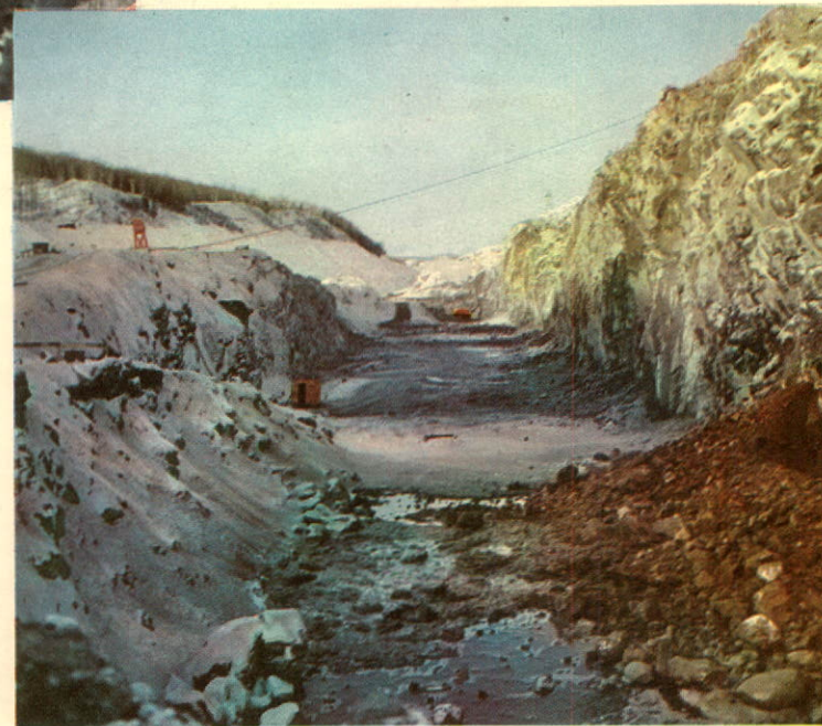
Excavation of the by-pass, a channel 1,500 feet long, 120 feet wide and 100 feet deep cut through bedrock, through which the river will be diverted during construction of the dam and powerhouse.
