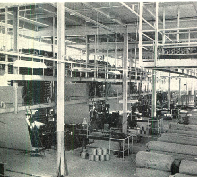
A carpet manufacturing plant recently established in our territory through the efforts of the Industrial Development Department.
