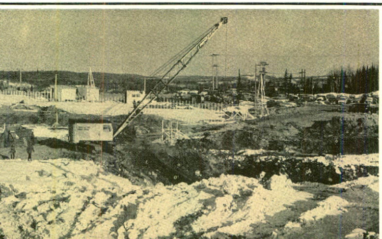
Excavating at Concentrator Area
