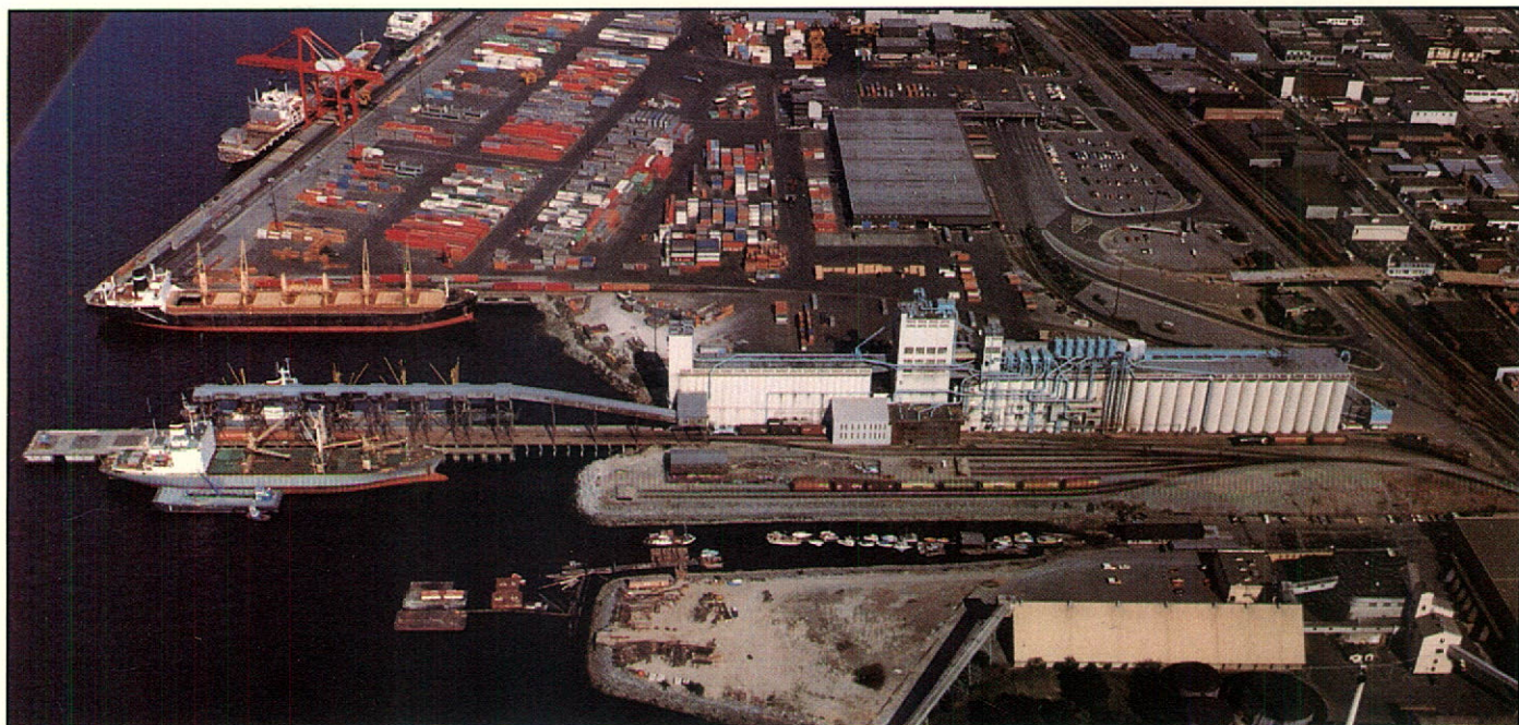
Vancouver terminal's west berth, damaged in mid-July, is now back in full operation. Shipments during the year were up 10.3 per cent over the previous year.
