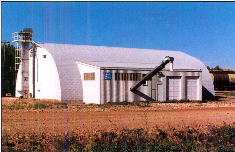
Hines Creek, Alta. new bulk blending fertilizer plant.
