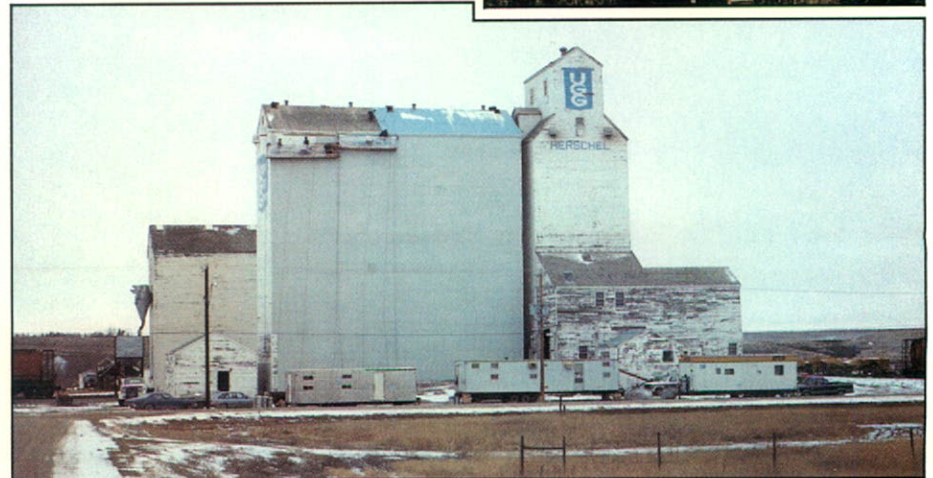
Herschel, Sask. elevator was upgraded and re-sited. Inset: Local Board Chairman Allan Coulter.
