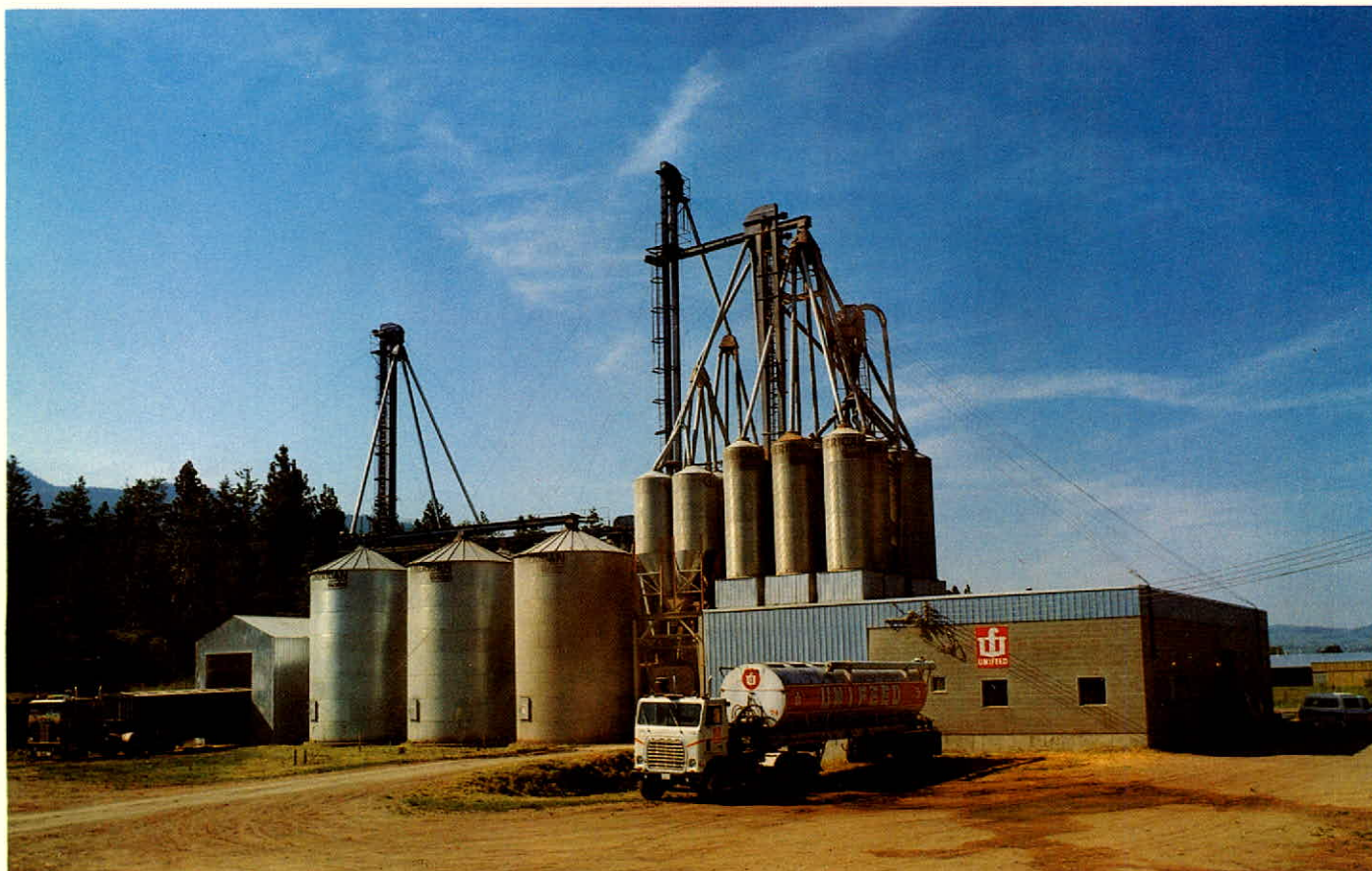
UGG has purchased the Armstrong Feed Mill in British Columbia.
