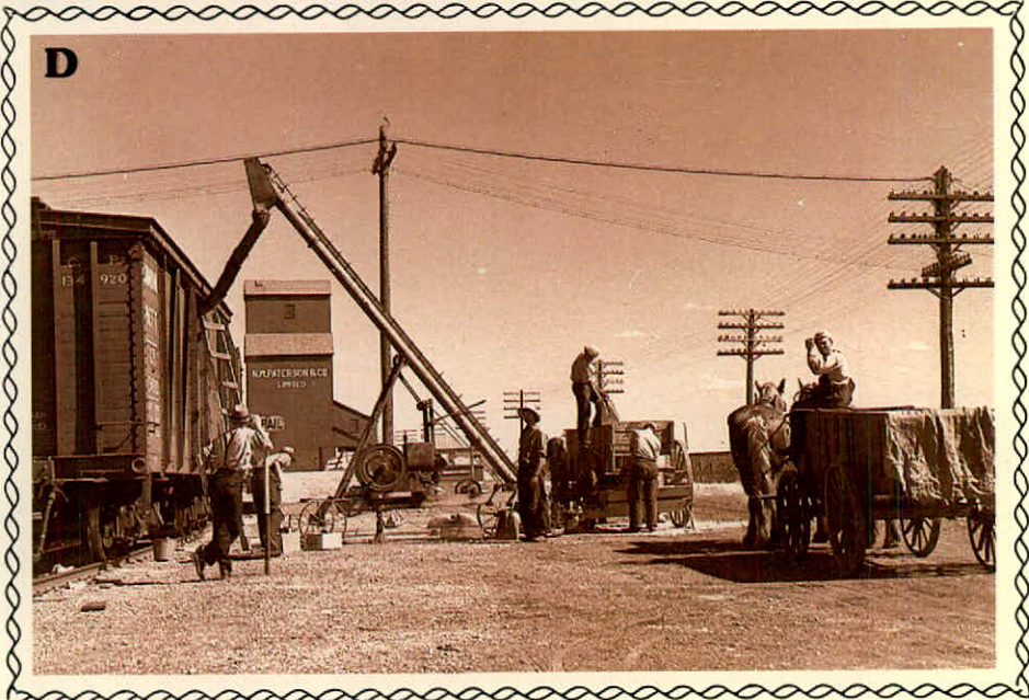
A new type receiving and loading facility (A) is being tested at Thorhild and at Bonnyville, Alta., to help reduce farmers' handling costs. At Thorhild, a 70-foot electronic scale weighs the largest trucks and then the grain is dumped into special auger hoppers (B & C) to be loaded into hopper rail cars. In the late 1930s, farmers loaded their grain into box cars with chain conveyors (D).
