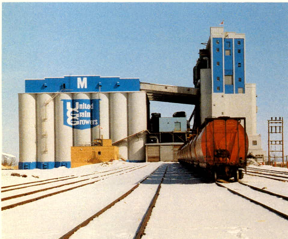
Modernization at Terminal M at Thunder Bay, Ont. was completed during the year.
