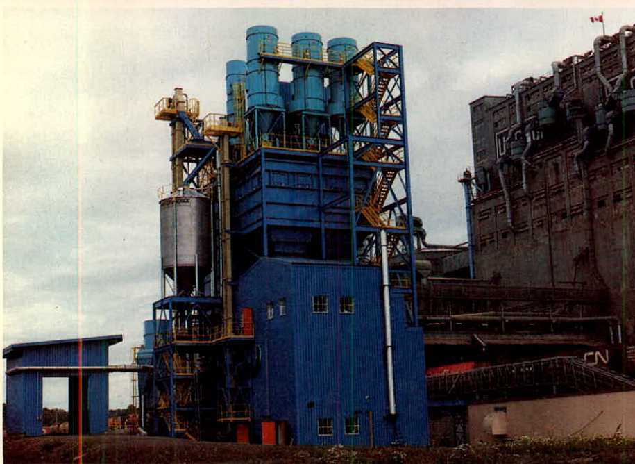
New pelleting plant at Thunder Bay, Ont. converts screenings and weed seeds into livestock feed. A truckload of screenings being weighed in (top left) and unloaded (top right).
