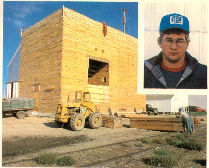
New elevator being built at Simpson, Saskatchewan. Gary Vanthuyne.
