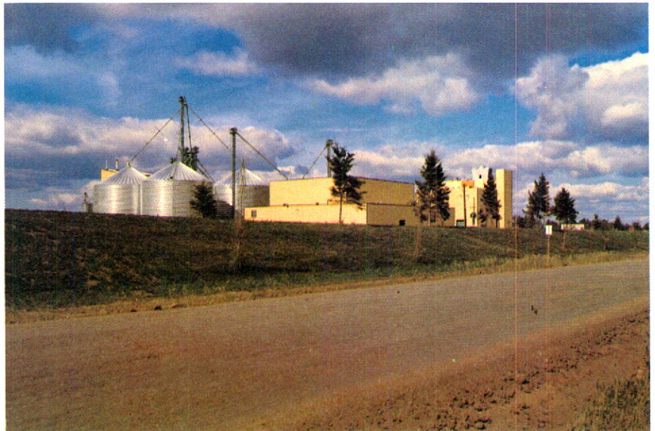
United Grain Growers now has one-half the modern United Oilseed Products plant at Lloydminster, Alberta. Its capacity is 180,000 tonnes a year.
