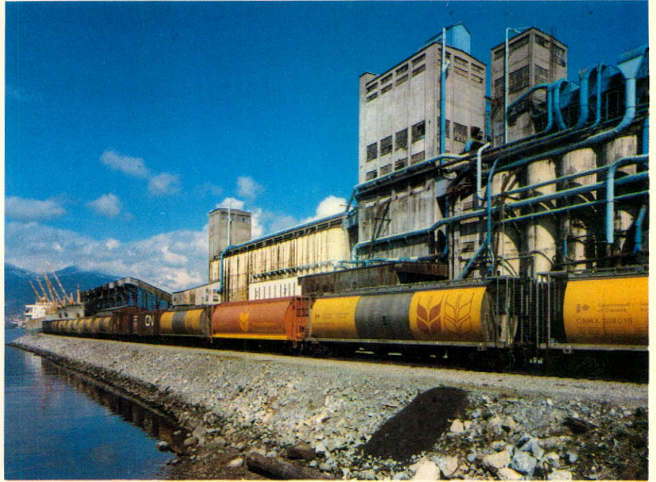
At the modernized Vancouver, British Columbia terminal, boxcars and hopper cars can be unloaded simultaneously. At the end of the loading gallery, a ship is being loaded with grain for Far East markets.
