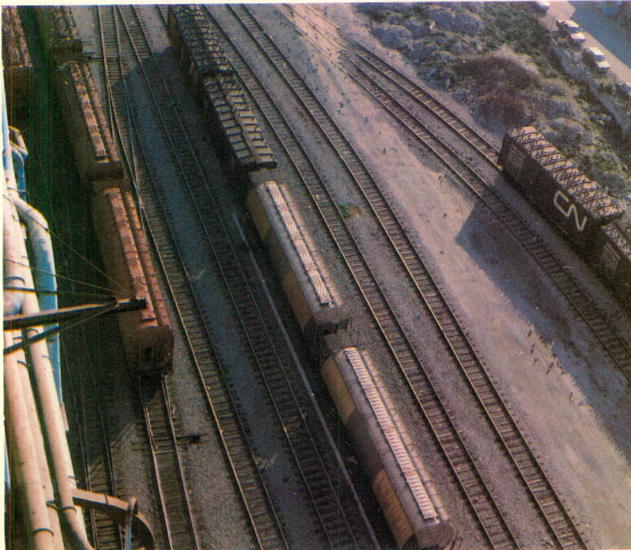
The UGG rail system at the Vancouver terminal has been completed. It can accommodate 85 hopper cars or 100 boxcars, almost triple that before modernization.
