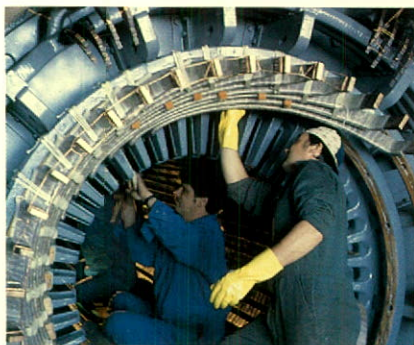
Replacing stator coils in electrical generators is a specialty of Westinghouse field service personnel.
