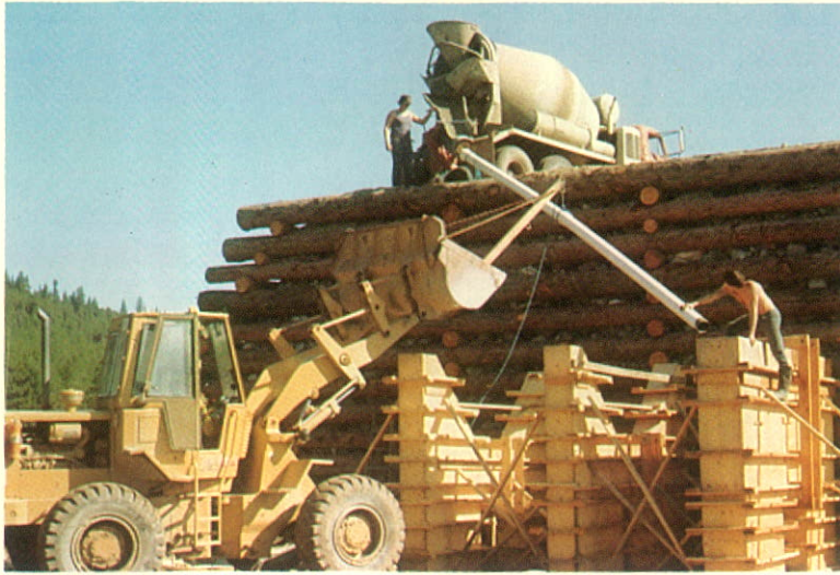
Placing concrete in foundation at Beaverdell.
