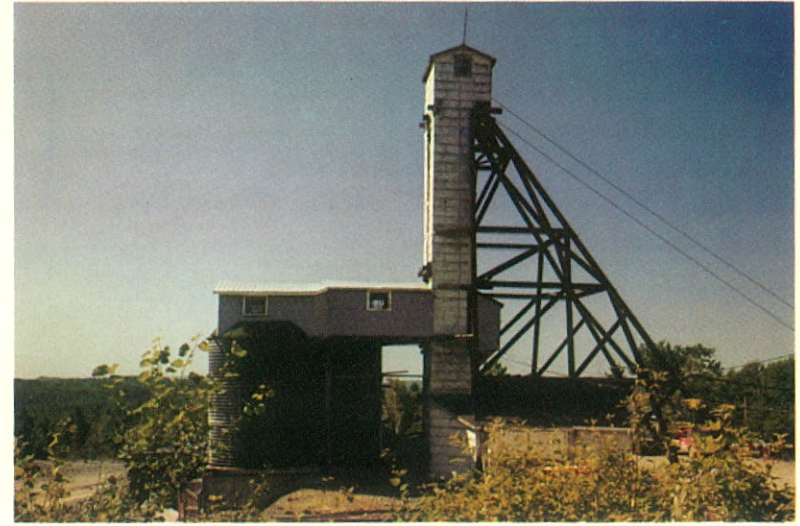
The Silverfields Mine headframe and ore storage bins.
