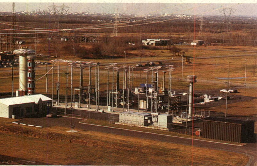
The high-voltage laboratory's underground-cable testing facility is now being used to assess 500-kV DC cables for the under-river crossing.
