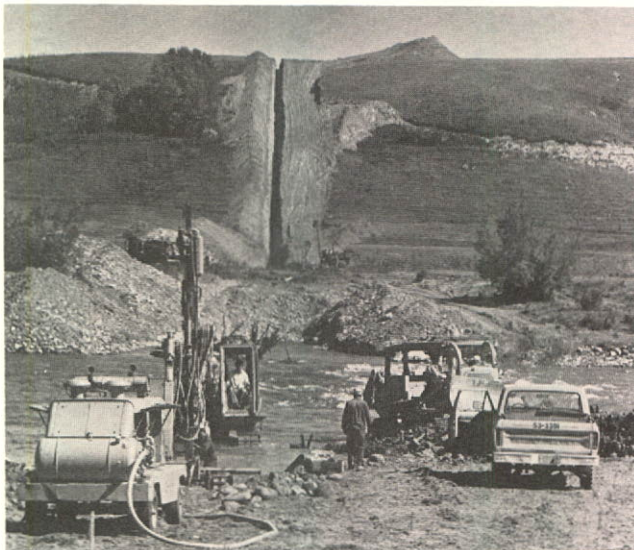
Drilling the ditch through the bed-rock of the Bow River, west of Calgary, in preparation for the installation of the pipe.
