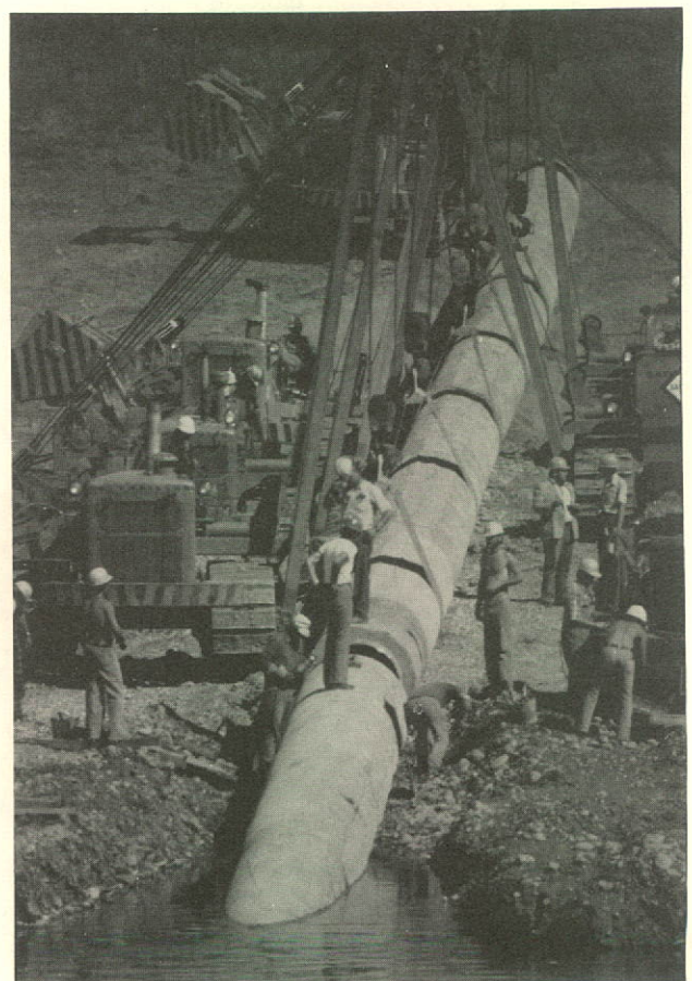
Sideboom tractors are used to submerge the first sections of pipe into the river trench during the crossing of the Bow River in Alberta. A bulldozer, anchored on the opposite shore is used to haul the pipe through the water with cables.
