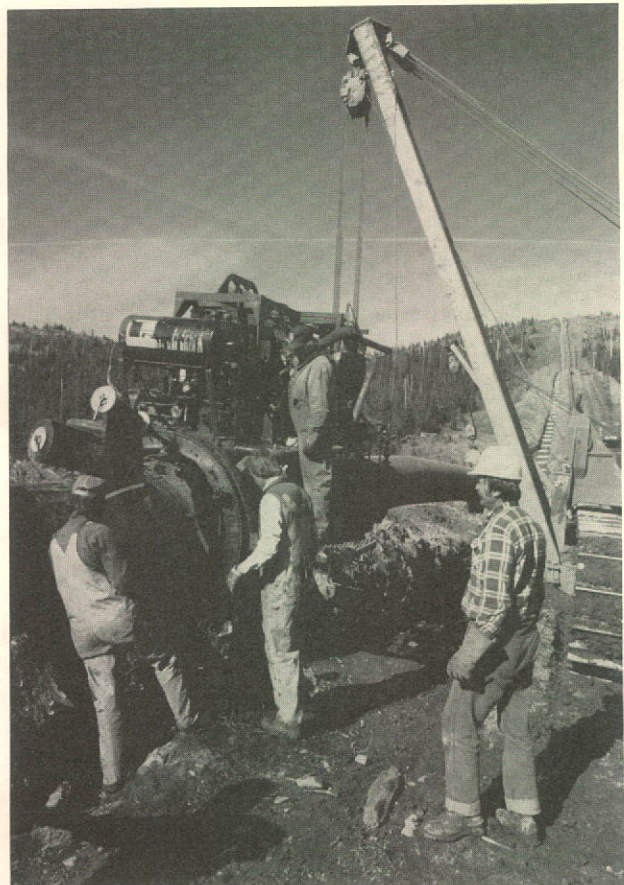
A coating and wrapping machine cleans the pipe, coats it with tar, and wraps it with polyethylene tape to protect the pipe from corrosion.
