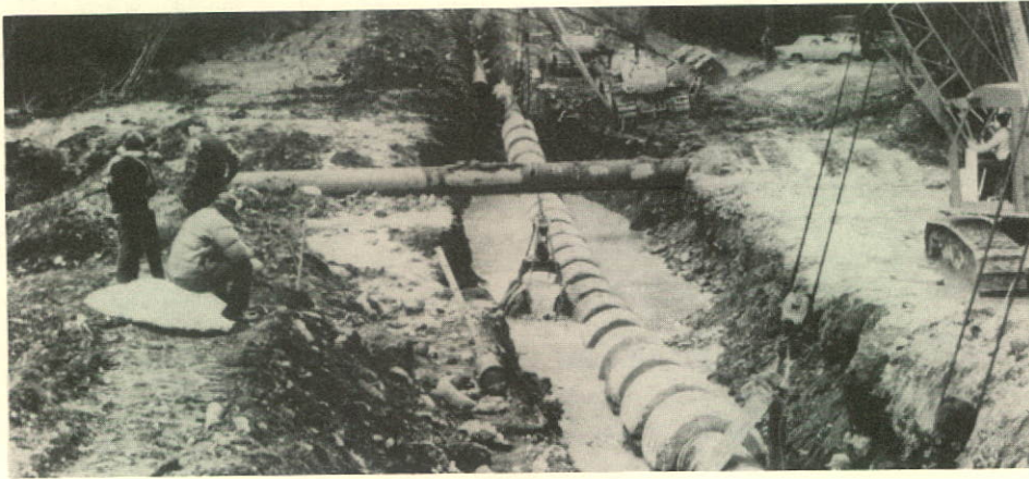
A flume is installed across the TeePee Creek in southern B.C. before the pipe is installed.
