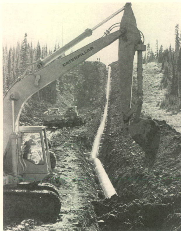
Backfilling the trench in the Flathead Ridge area of Southern B.C.
