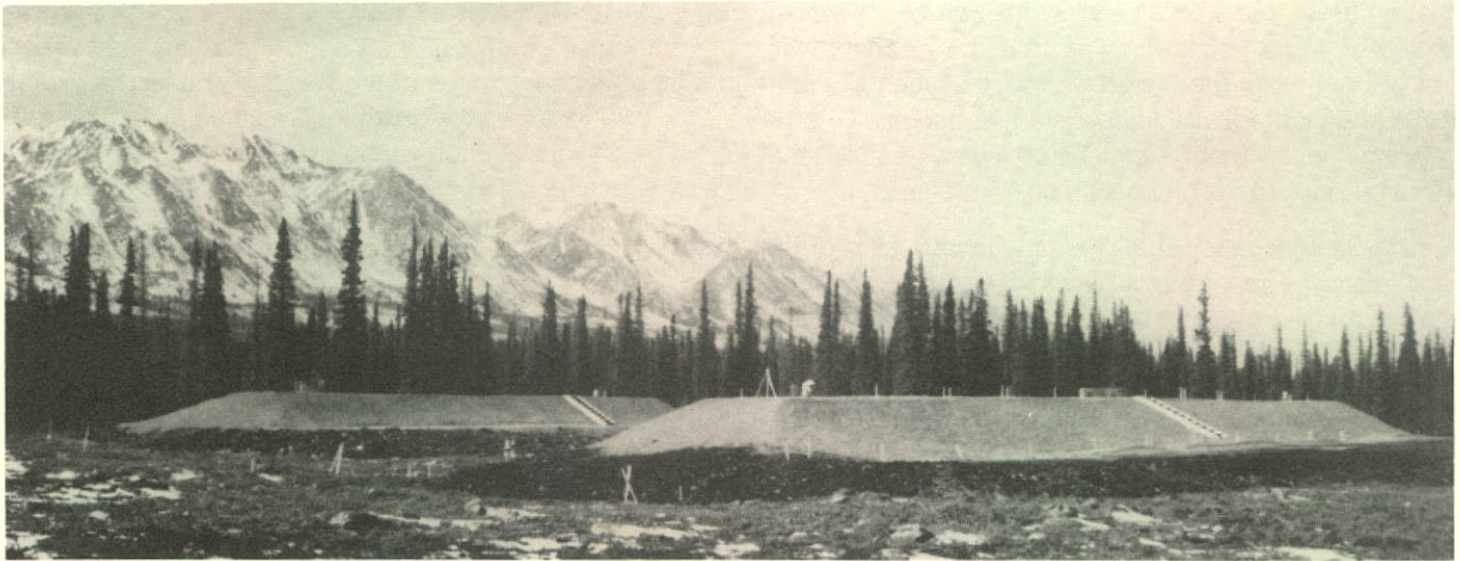
At the Quill Creek test facility, undertaken by Foothills (South Yukon) Ltd. to determine the feasibility of constructing and operating a pipeline in areas of discontinuous permafrost, pipe is installed in embankments that measure approximately 3.3 metres (10 feet) above the ground. The embankment mode consists of a gravel pad on which an insulation bed and pipe are laid and then covered with gravel. For the purposes of testing thaw settlement, pipe is also buried in the conventional manner.
