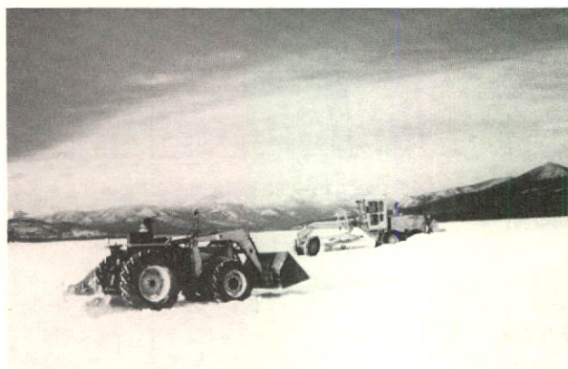
As part of the Quill Creek test program, an experiment was carried out using ice as a protective road-bed over permafrost. Shown above, a large roto-tiller attached to a farm tractor harvests ice chips from Kluane Lake for use in access road construction.
