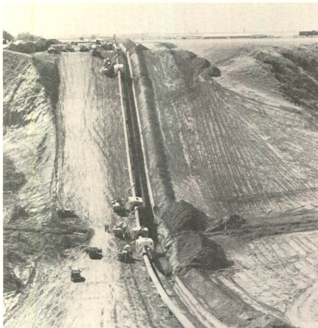
Automatic welders move down the 45-m (140 ft.) deep west bank of Irishman's Coulee in eastern Alberta.
