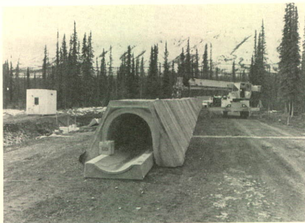
Experimental pipe installation in aboveground concrete restrained mode at Quill Creek test facility in Yukon. The pipe is placed on an insulated workpad and covered by precast concrete for protection and to provide restraint of the pipe against vertical and horizontal movements due to temperature and pressure changes.
