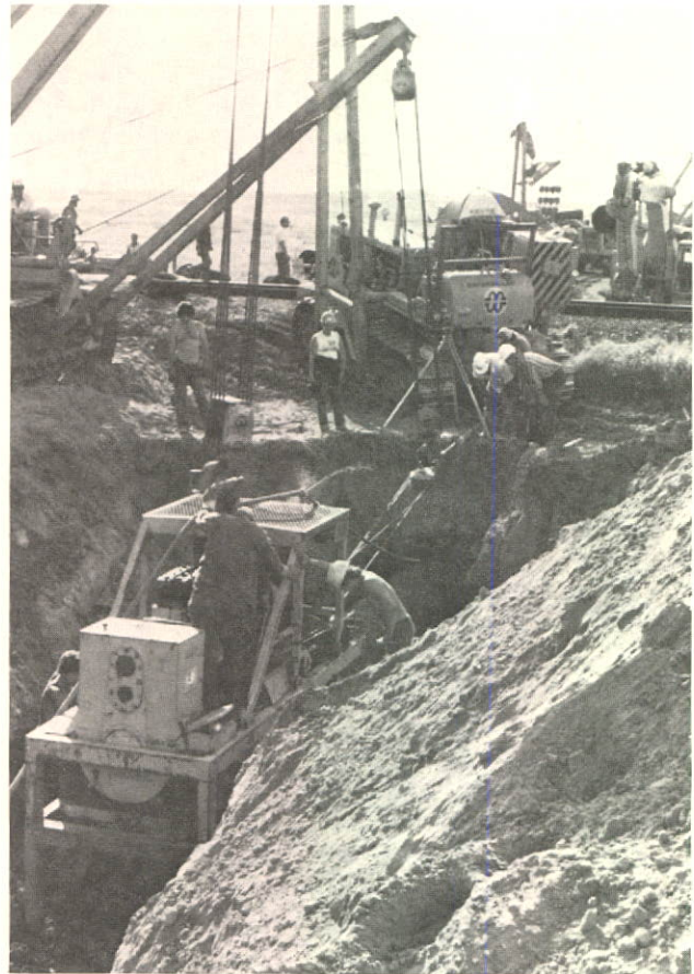
Pipe is installed under a railroad near Piapot, Saskatchewan using a "slip bore". Powered by the machine in the foreground, an auger inside a length of pipe bores a tunnel under the railroad. The pipe is then pulled or "slipped" out and the "carrier" or permanent piece of pipe is inserted.
