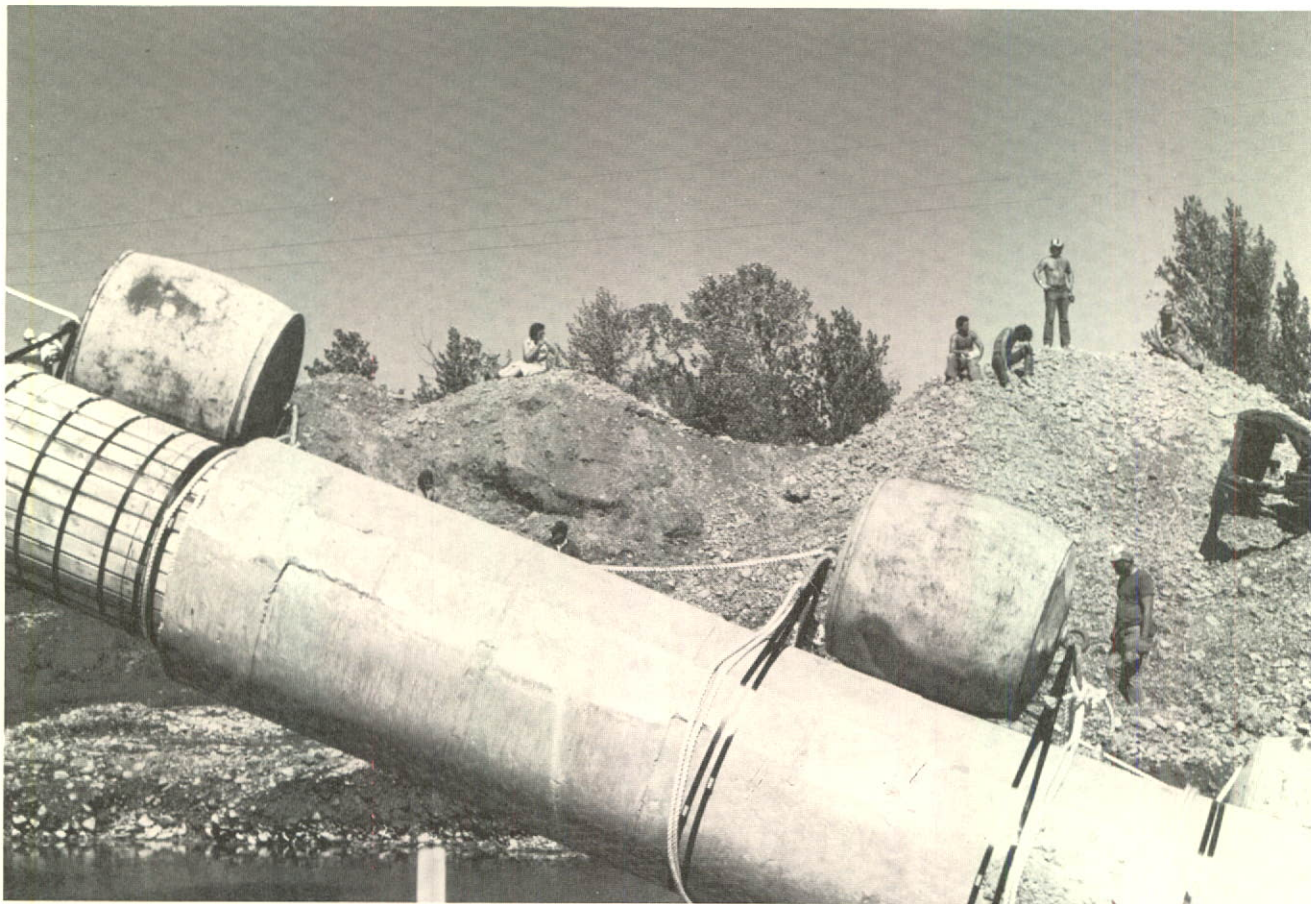
In preparation for a major river crossing, floats are attached to the pipe to maintain buoyancy while pulling the pipe across the body of water.
