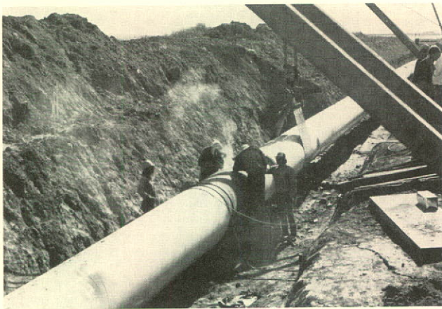
The final tie-in weld, completed on August 17, 1982, south of Beiseker, Alberta, wraps up construction of the Eastern Leg of the pipeline in Canada.
