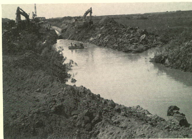
Foothills inspectors check the depth of the ditch for the pipeline crossing of Serviceberry Creek along the Eastern Leg in Alberta.
