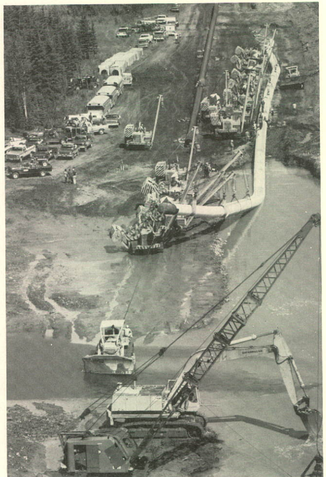
Construction crews prepare to lower the pipe into the river bed during Eastern Leg construction.
