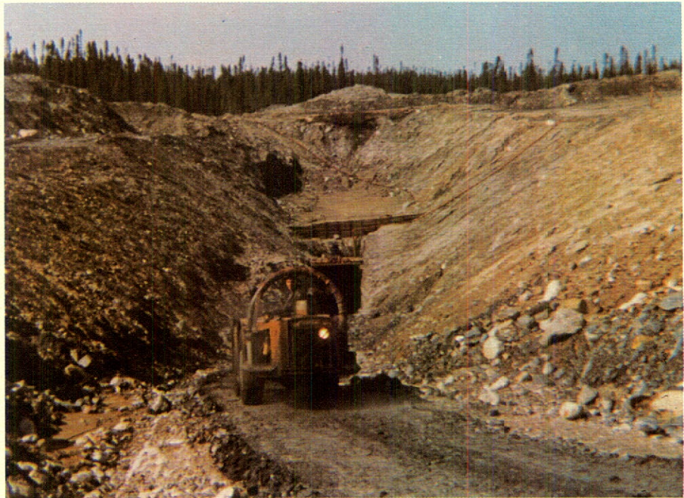
Portal opening at the Perch River property.
