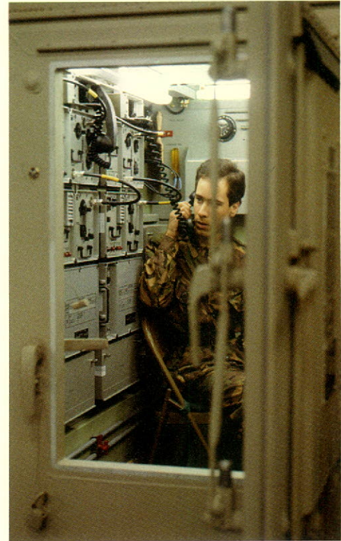
Transportable shelters house fully integrated CMC tactical communications systems.
